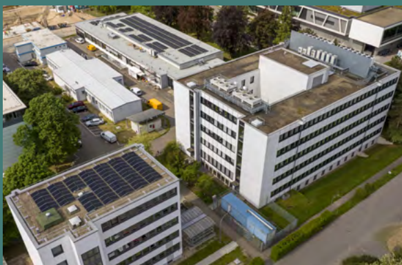
Figure 21: Photovoltaic systems FIZ Karlsruhe
